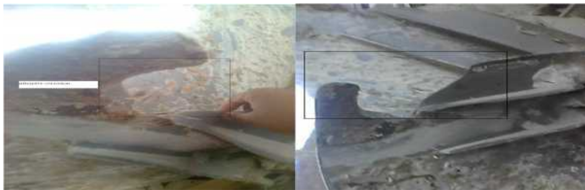
Fig (1): Corrosion of ferralium in agitator reactor.
