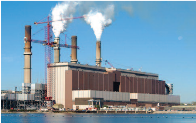
Gibson Station is now Duke Energy's largest power plant. It is a five-unit facility that was built between 1976 and 1982. Unit 5 is co-owned by Wabash Valley Power Association and Indiana Municipal Power Agency. All five units have sulfur dioxide scrubbers.
