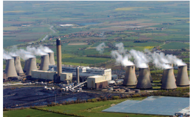
Drax Power Station is the largest generating station in the UK. Pollution control systems are installed in all units, although the station has been partially converted to use biomass instead of coal.
